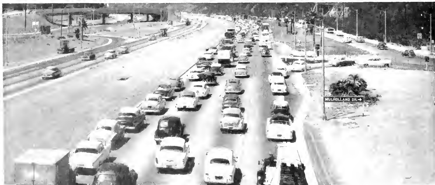
View looking northerly along Hollywood Freeway from Pilgrimage Bridge showing Highland off-ramp overcrossing center left. The cleared space between the two main freeway roadways is the strip of land 48 feet wide recently acquired from the Pacific Electric Railway after abandonment and track removal. This additional area will be available for future freeway improvement as needed.
